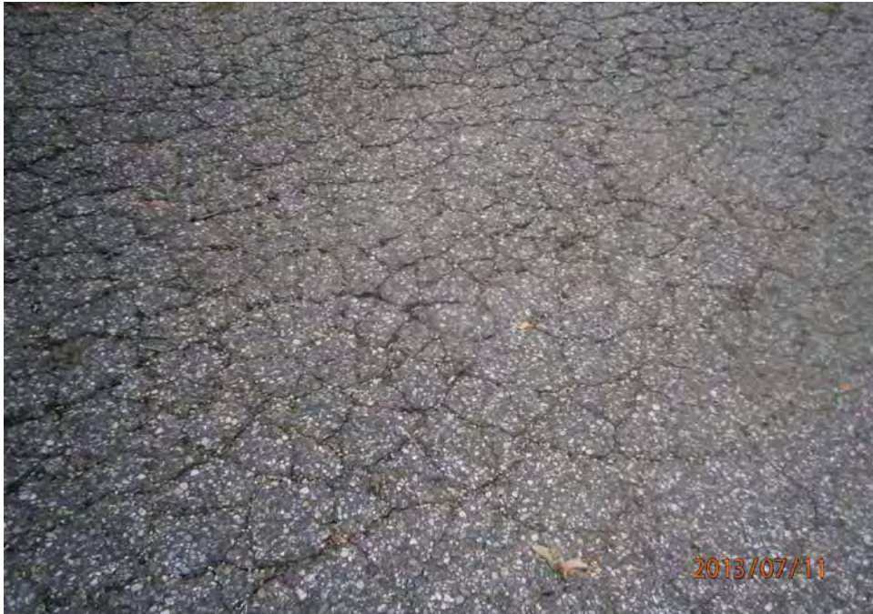
1. Asphalt parking area; cracked
