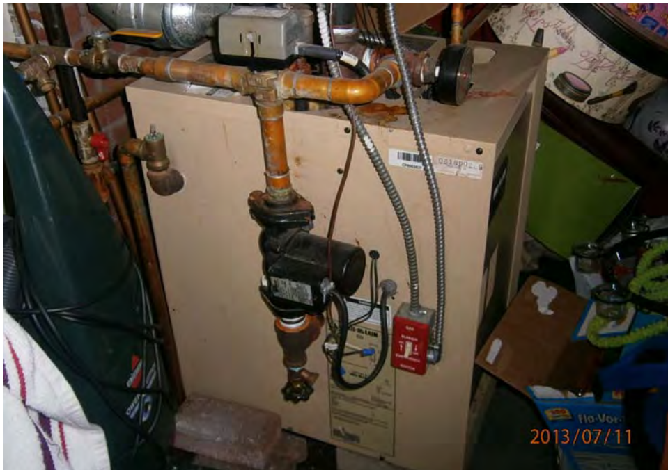
23. Typical unit boiler
