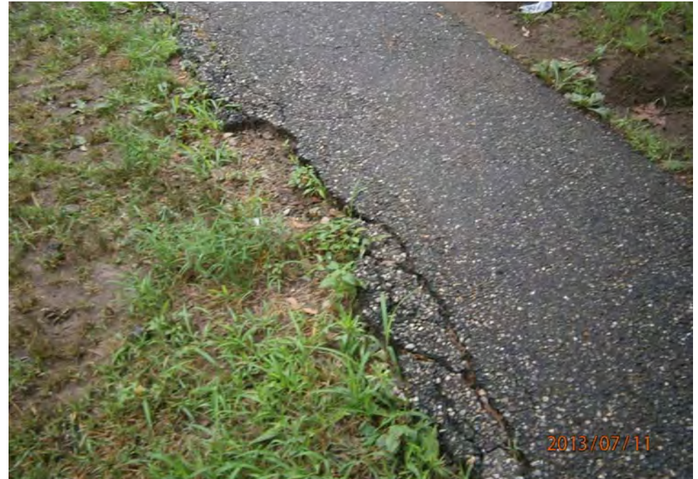
2. Asphalt walkway; spalled and damaged
