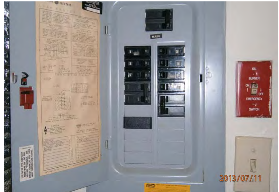
24. Unit circuit breaker panel
